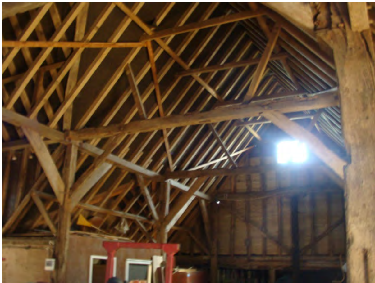
Picture 1.6 Interior of reconstructed barn being that to the south east of Upper Farmhouse. Original structure burnt down in 1980.
