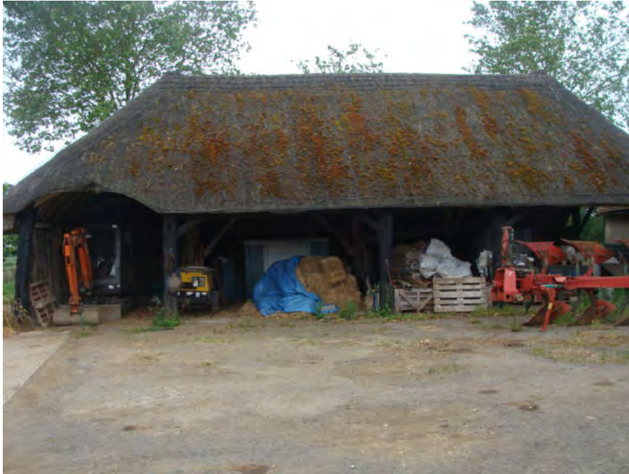
Picture 1.7 Single storey open fronted curtilage listed cart lodge to south west of Upper farmhouse.
