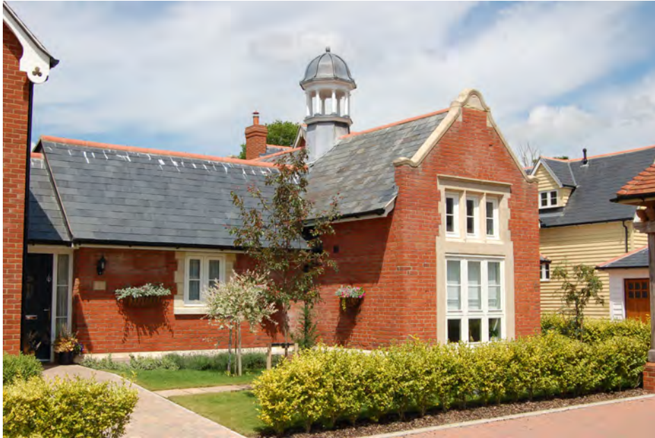
Picture 1.14 The former electricity generating house from the Hargrave Park estate, now converted to residential use.
