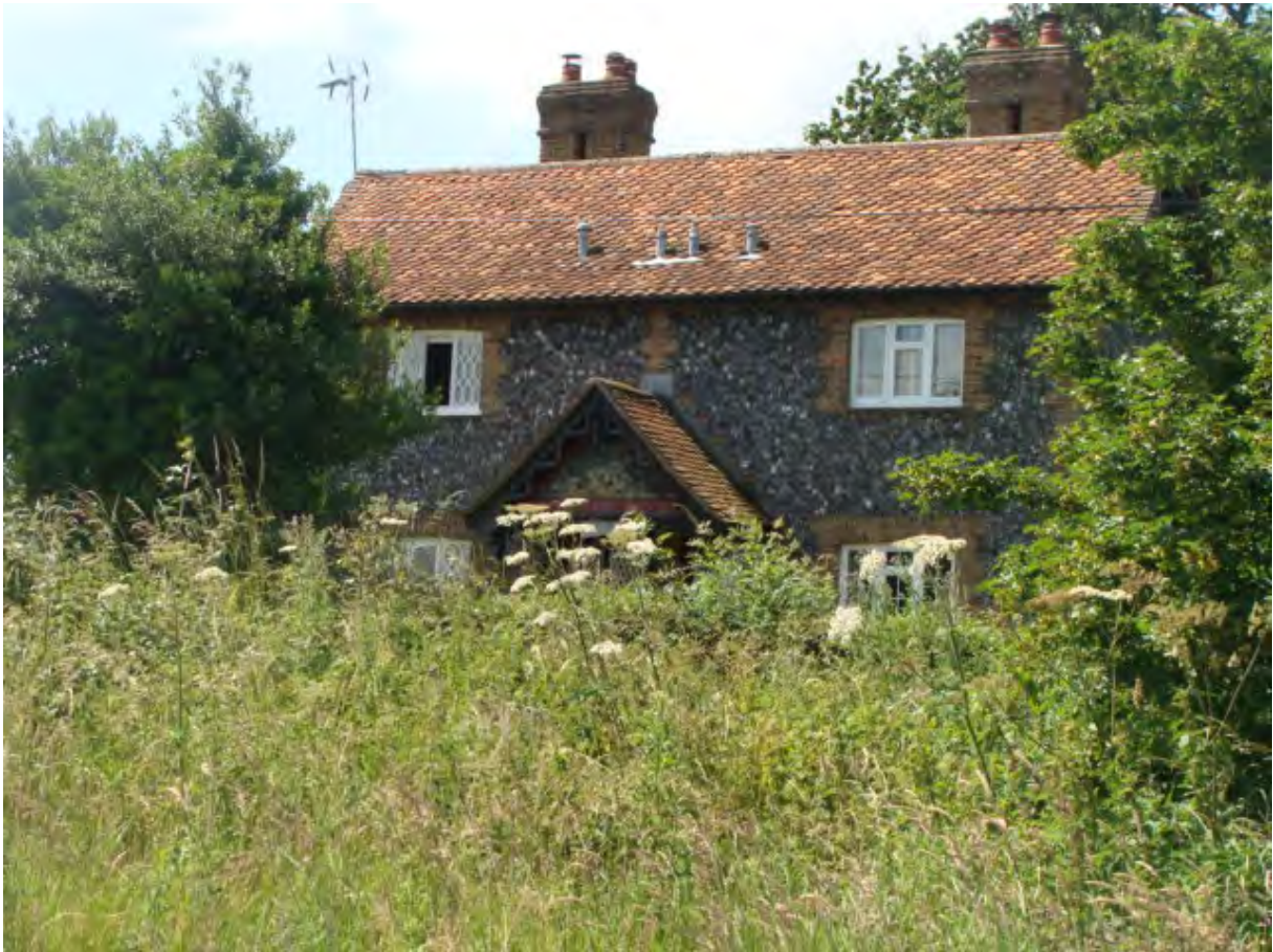
Picture 1.5 Estate Nos. 58 and 59 (Stone Cottage). Delightful typical mid 19th century estate cottage.
