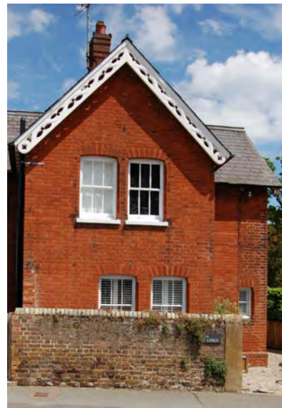
Picture 1.5 Decorative barge boards employed to dramatic effect under a slate roof on West Lodge - a building formerly associated with the Hargrave Park estate.
