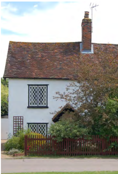
Picture 1.4 Clay tiles, white-washed plaster and distinctive diamond pane windows behind a simple picket fence on Laundry Cottage.
